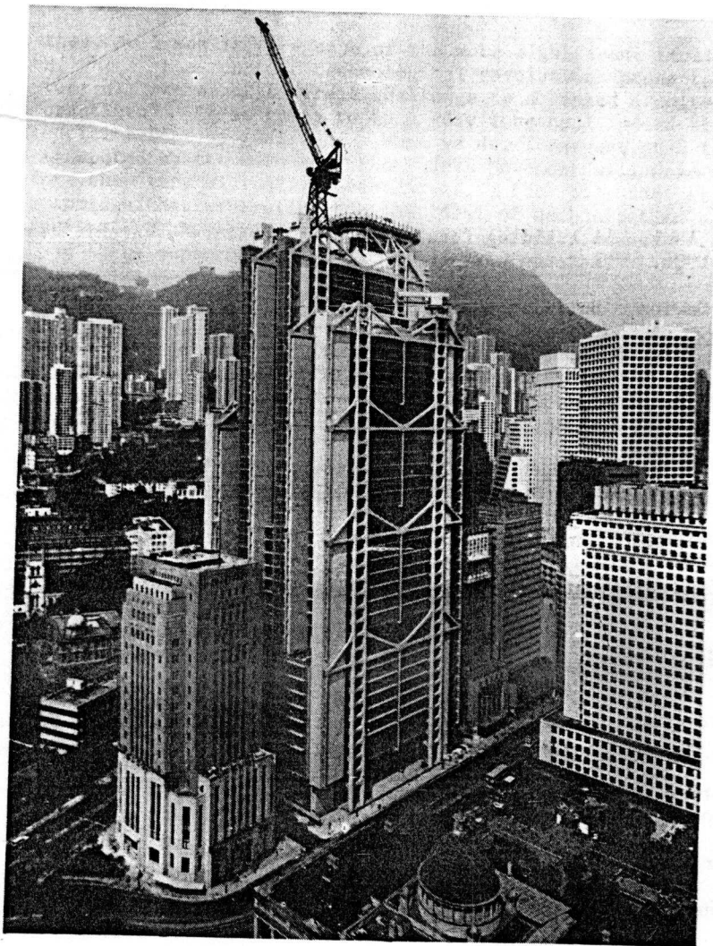
The Hongkong and Shanghai Bank headquarters, Designed by Foster Associates. State of the art computerized presses and robot welders were used in the manufacture and assembly of the aluminium cladding, made up of thousands of separate pieces of different size and shape.
